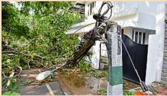
An electric pole in Sadashivanagar broke after a tree branch fell on it.
